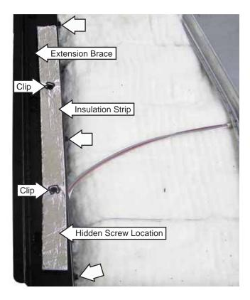
6. Remove 1/4-in hex-head screw that attaches the back of the extension brace to the range.
