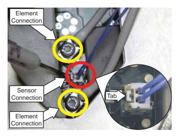
Note: On the 11-in. element, the choke must be removed and transferred to the replacement element. The choke must be attached at the same location on the wires and secured with a plastic wire tie.
