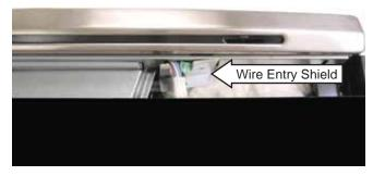
3. Pull the cooktop wiring thru the wire entry and disconnect the 2 wire harnesses that connect the cooktop assembly to the range.
