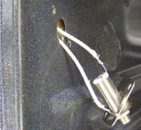
2. The outlet and wiring can be pulled out approximately 1½”.
