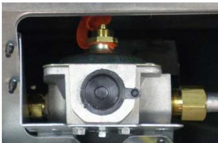
The regulator has an adjustment for converting the range from natural gas to propane (LP). The adjustment screw is marked to show which way is up for natural gas or propane (LP).
