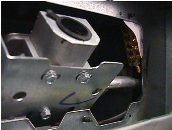
The propane (LP Gas) instructions are attached to the back of the range. Inside, near the gas valve, is a set of LP orifices for the conversion.
