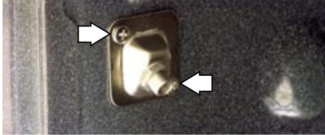
The outlet and wiring can then be pulled down from the oven wall approximately 1½ inches.
