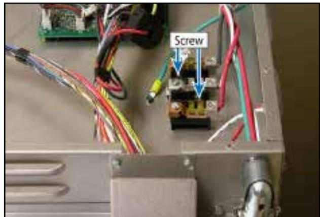
5. Repair or replace terminal block as necessary.
