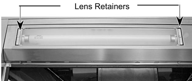
4. Slide the fluorescent lamp lens to either end of the holder and remove it from the holder tabs.
