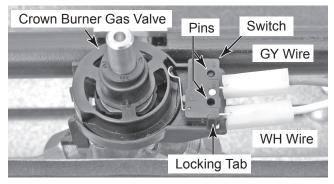
e) Disconnect the two 1/2<sup>"</sup> gas line fittings from the gas valve.
